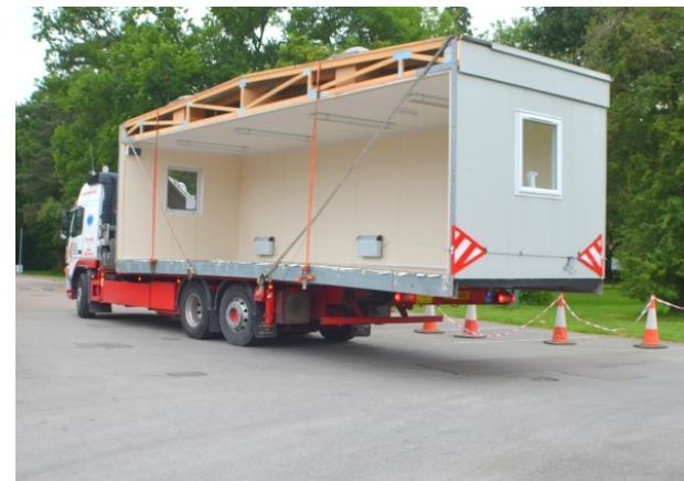
The modules are delivered in sequence and offloaded by mobile crane.
