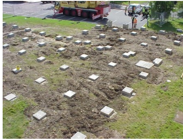
The foundations are formed by concrete slabs laid on a levelled site.
